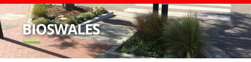
Much like rain gardens, bioswales also collect and filter runoff, but instead of using native plants alone, bioswales channel stormwater into a trough filled with multiple layers of vegetation, compost, mulch or rubble. They are often located near roads or parking lots to capture the associated runoff. Bioswales have been found to reduce surface runoff by almost 99% and are relatively inexpensive and easy to implement.
